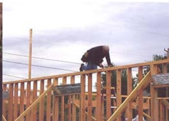
Tie those walls together
