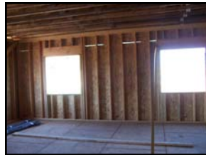
Walls studded in with 9 foot ceilings and 2 x 6 outer frame studs
