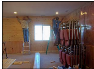
Bob and Skip hang wood on walls
