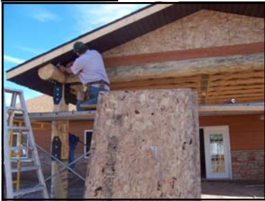
Glen installs siding
