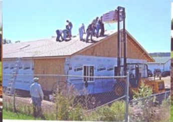
Roof sheeting time
