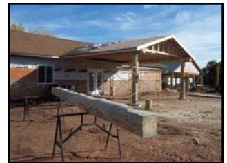
No maintenance siding and rock Insulation installed Overhang up and ready for a major log install
