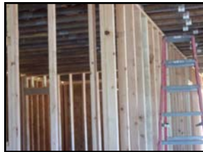
Walls studded in with 9 foot ceilings and 2 x 6 outer frame studs
