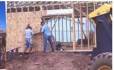
Lets get these walls covered
