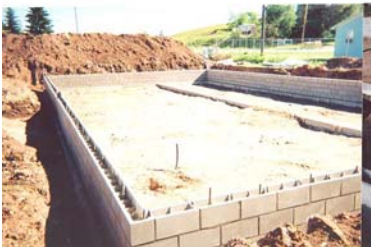
Here's the floor assembly
