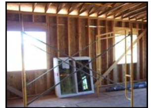
Walls studded in with 9 foot ceilings and 2 x 6 outer frame studs
