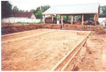
Floor goes on over floor joists
