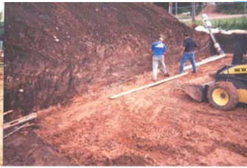
Foundation forms installed
