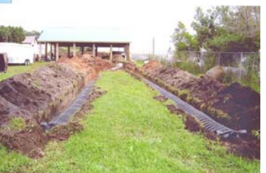
Drain field trench
