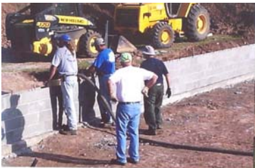
It's time to put floor joists in
