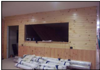
Getting ready to lay floor
