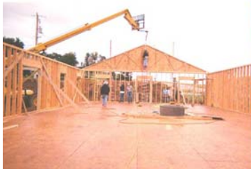
Starting to put up the roof trusses
