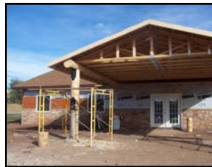
No maintenance siding and rock Insulation installed Overhang up and ready for a major log install
