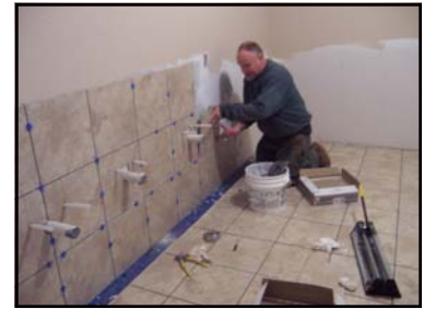
Erv puts tile on walls
