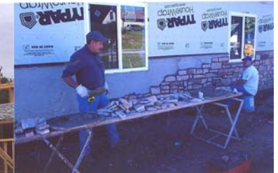
Steve works on the rock lower wall covering
